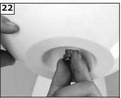
Install light plate over all thread and use nut provided to secure in place.
